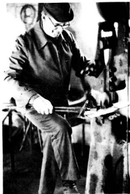
Ralph Pippin at the triphammer sharpening ploughshare.
